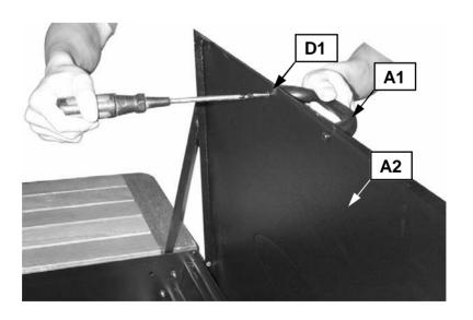
Attach the lid handle (A1) to the lid (A2) using the handle bolts (D1).
